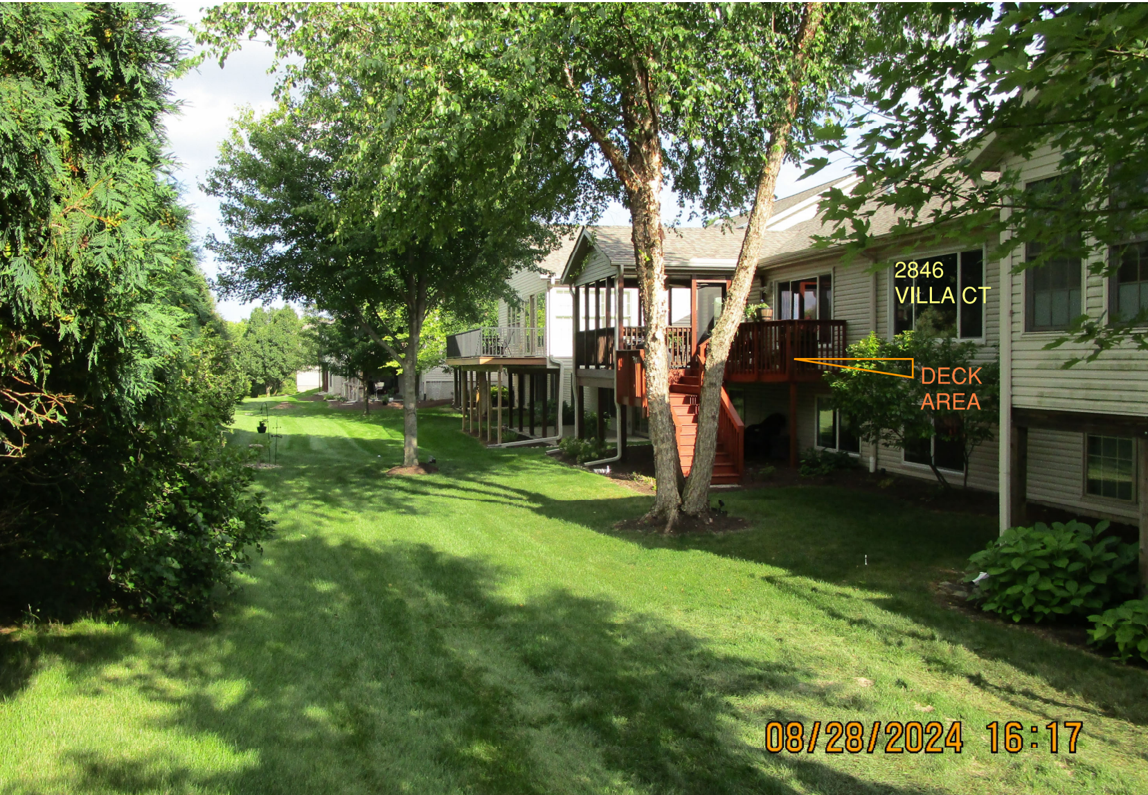
2846 DECK BUILD OUT LOCATION
